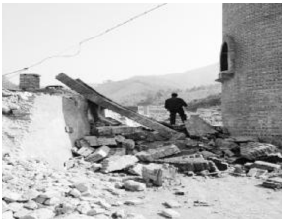
Figure 2 Before the removal of flue
